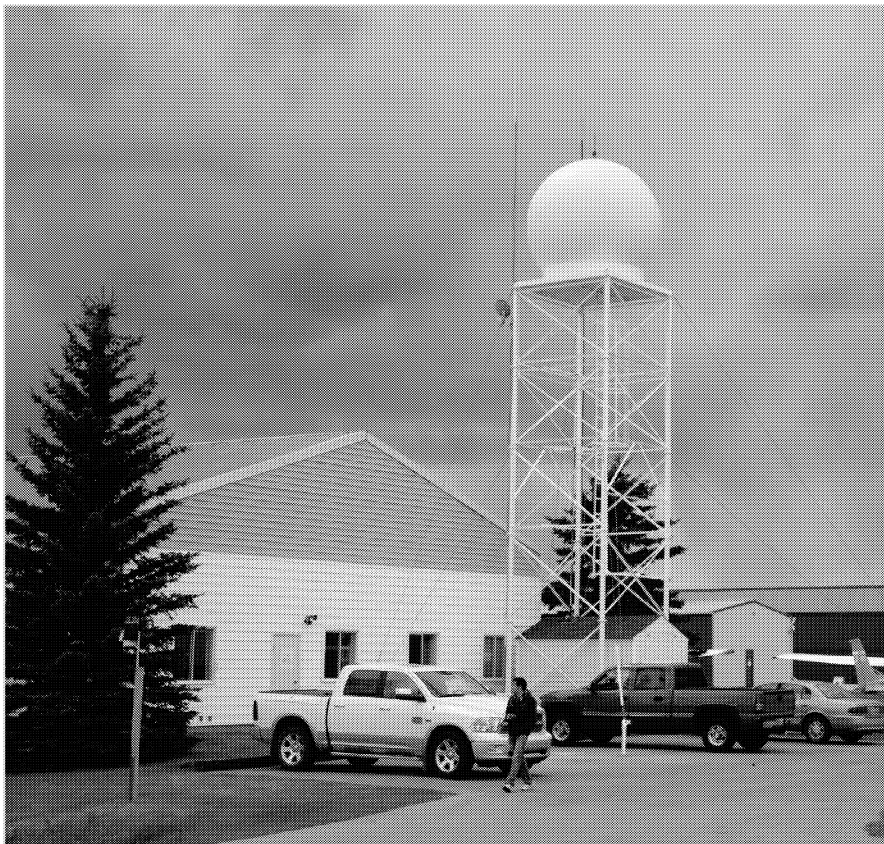
Fig. 15. The WMI project Operations Centre is located at the Olds-Didsbury Airport, about 70 km (44 miles) north of the Calgary Airport, roughly halfway between the project's most important cities: Calgary and Red Deer. The radar antenna is housed within the dome, and the transmitter and receiver in the shed at the tower base. Operations are conducted from within the meteorological office housed within the adjacent hangar. (WMI photograph by Bruce Boe.)
